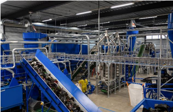
Figure 51 – FastFeetGrinded line in Heerhugowaard (NL)
